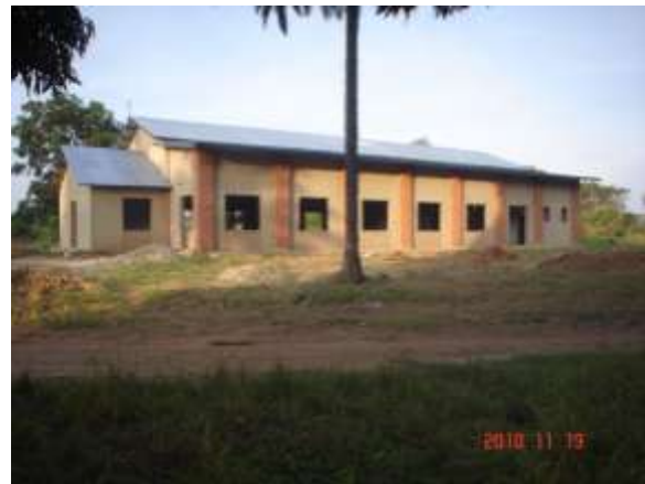
Cathedral Construction in progress
